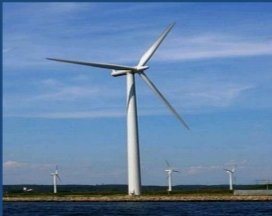
Horizontal Axis Wind Turbine
